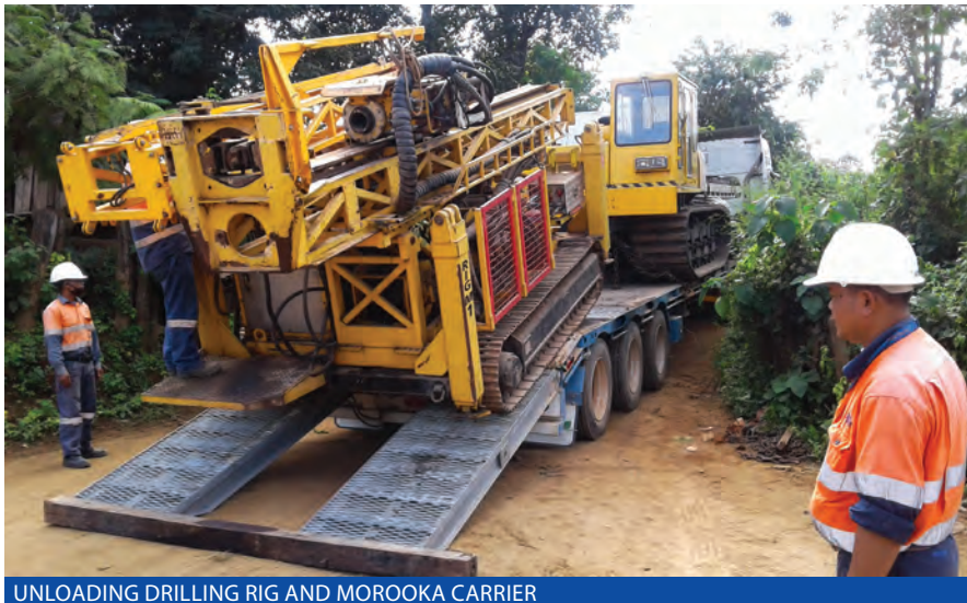
UNLOADING DRILLING RIG AND MOROOKA CARRIER
