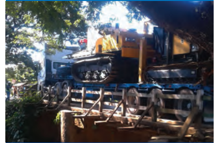
CROSSING ONE OF MANY WOODEN BRIDGES
