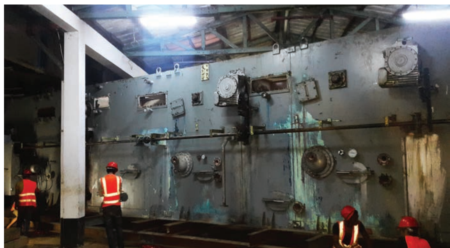
BOTTLE WASHER BEING MANOEUVRED BY SKATES FROM ITS ORIGINAL LOCATION
