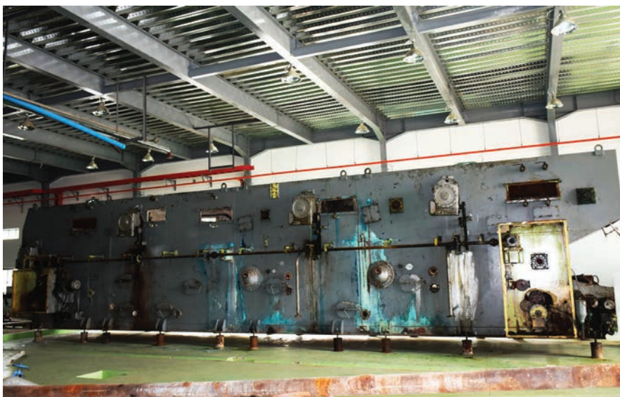
BOTTLE WASHER IN POSITION AND READY FOR COMMISSIONING
