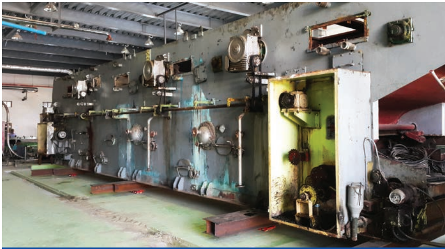
THE BOTTLE WASHER BEING LEVELLED AT ITS FINAL LOCATION
