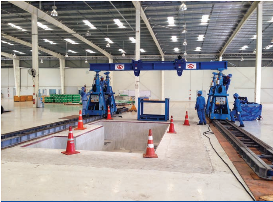
TEMPORARY GANTRY CRANE ERECTED FOR THE INSTALLATION OF THE PRESS
