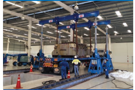
BED SECTION LIFTED FROM CEA TRAILER
