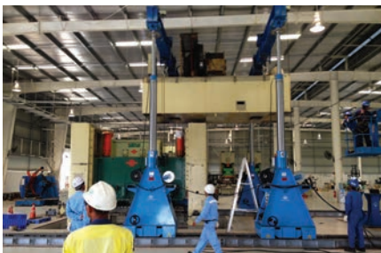
CROWN SECTION BEING MOVED INTO PLACE
