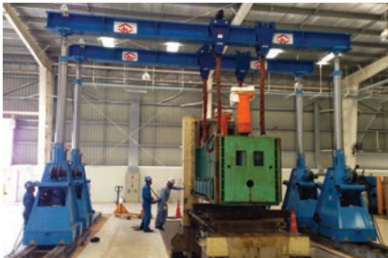
PRESS SLIDE MOVED INTO PLACE
