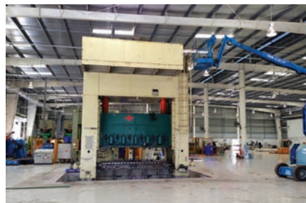
COMPLETED PRESS INSTALLED
