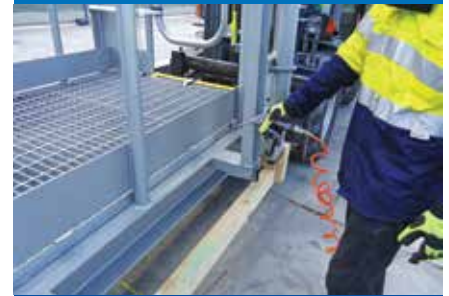
RESIDUAL WATER & DUST CLEANED AWAY
