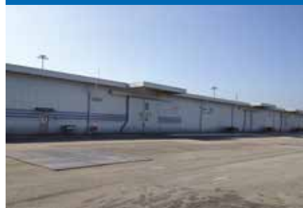
COMPLETED WAREHOUSE AT FTZ1
