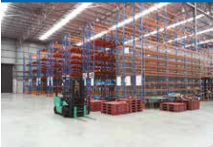
INTERNAL RACKING FACILITIES
