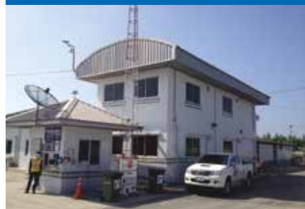
OFFICE BUILDINGS FABRICATED BY CEA
