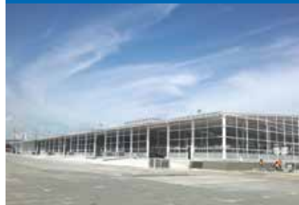
WAREHOUSE 1 UNDER CONSTRUCTION
