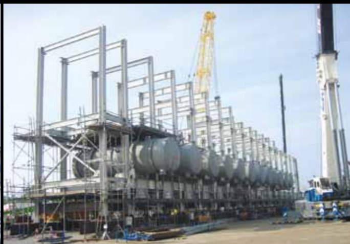
14 x 100t tanks installed using CC2400 in 6 days
