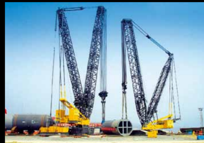
LR11350 & LR1750 tandem lift 800t pressure vessel.
