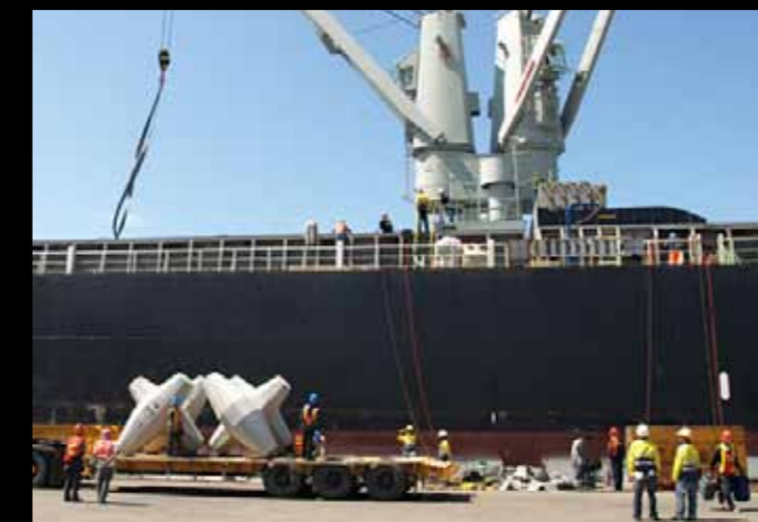
Loading vessel of Core-Loc's bound for Sino Iron Project
