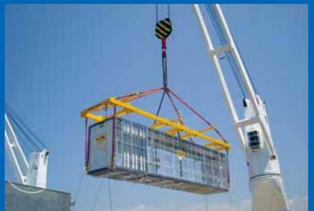
Lifting and loading of 20t module onto the vessel
