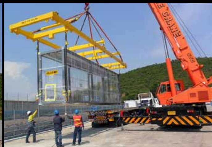
Loading of accomodation module for the Gorgon Project
