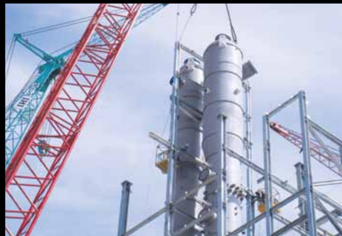
Two 148t column lifted safely into position
