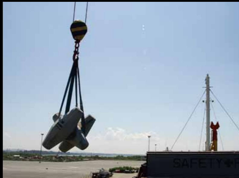
Loading of 385 units of 20t Core-Loc's
