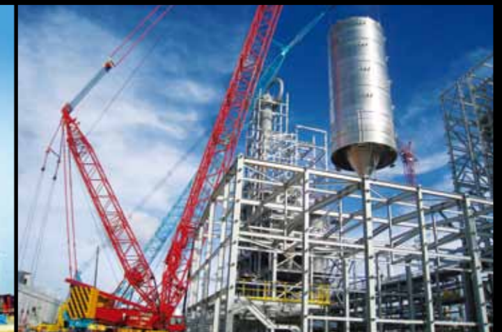
30m x 16m diameter silo using CC2800 with super lift
