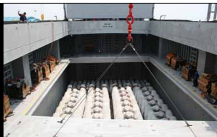
Stowage of Core-Locs on vessel tank top
