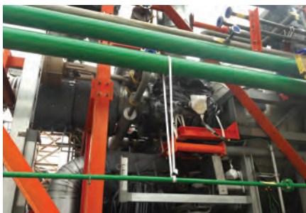
STEEL SUPPORTS INSTALLED BY CEA
