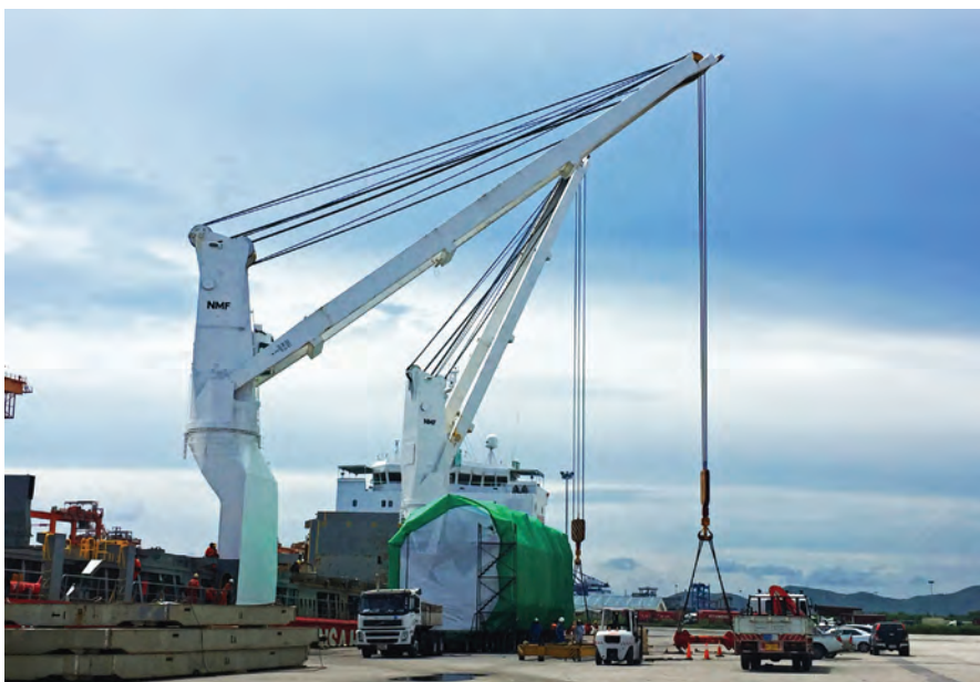
LOADOUT OF THE MODULES AT LAEM CHABANG PORT, CHONBURI
