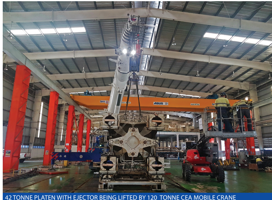
42 TONNE PLATEN WITH EJECTOR BEING LIFTED BY 120 TONNE CEA MOBILE CRANE
