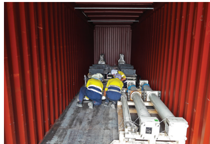
WOODEN CHOCKS BEING INSTALLED
