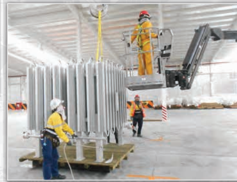
An Elevated Work Platform (EWP) is used to help clean a gas heat exchanger
