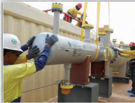
A pressure evaporator is carefully lowered and secured into an open top container
