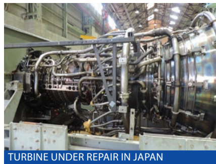
TURBINE UNDER REPAIR IN JAPAN
