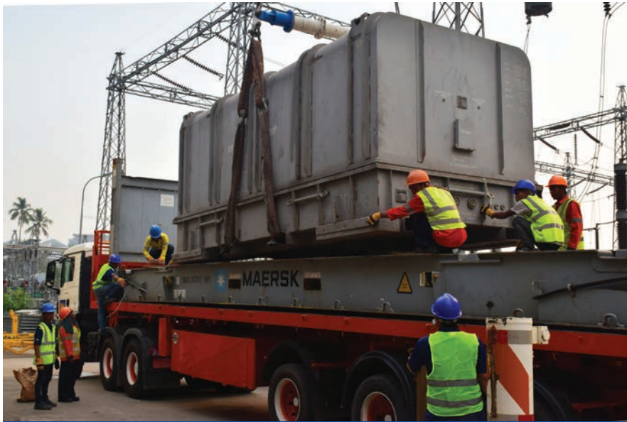
TURBINE UNIT LIFTED AND MANOEUVRED INTO PLACE BY THE CEA PROJECT TEAM
