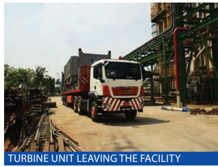
TURBINE UNIT LEAVING THE FACILITY
