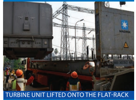
TURBINE UNIT LIFTED ONTO THE FLAT-RACK
