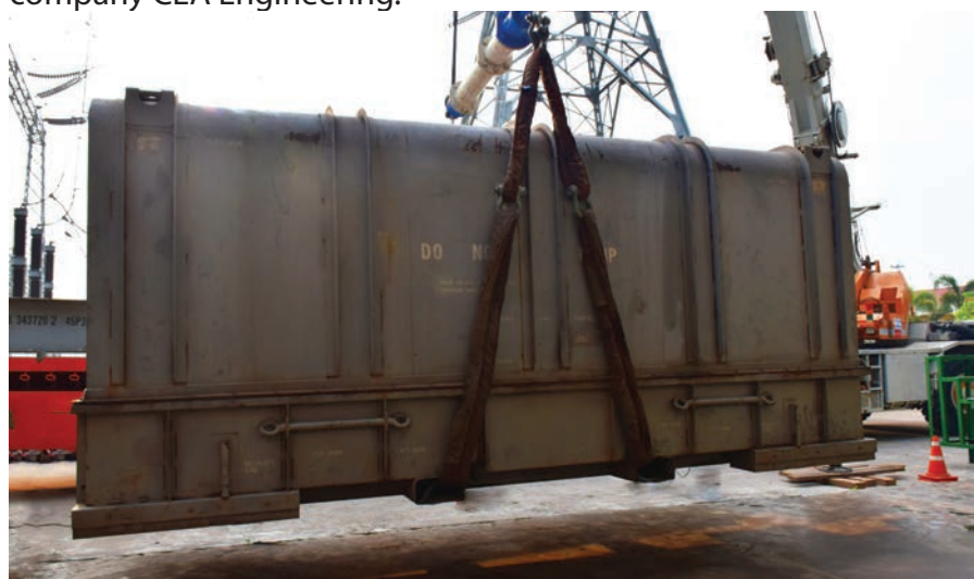
A 50 TONNE MOBILE CRANE WITH SURELIFT SPREADER BEAM LIFTS THE TURBINE UNIT
