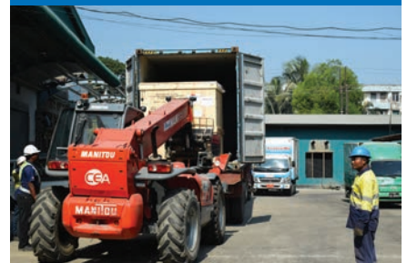
TELEHANDLER UNLOADING CONTAINERS
