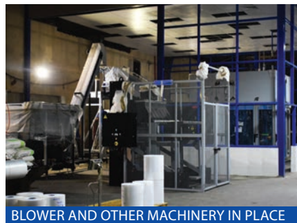
BLOWER AND OTHER MACHINERY IN PLACE
