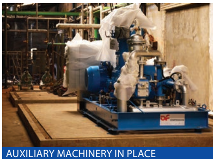
AUXILIARY MACHINERY IN PLACE
