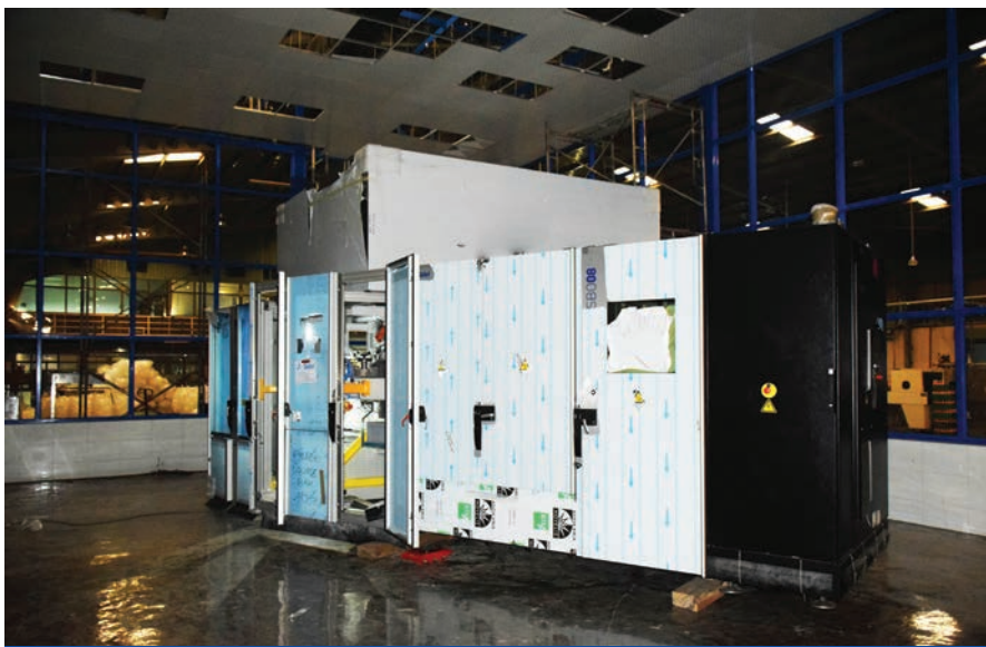
MAIN PARTS ASSEMBLED IN OPERATIONAL LOCATION AND AWAITING FINAL INSTALLATION
