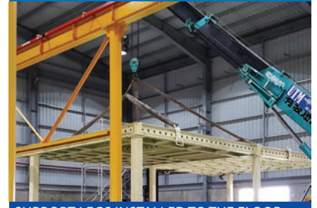
SUPPORT LEGS INSTALLED TO THE FLOOR
