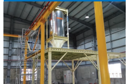
RAW MATERIAL HOPPER INSTALLED
