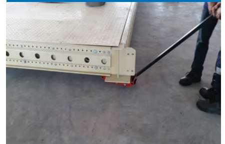
MEZZANINE FLOOR MOVED BY 12T SKATES
