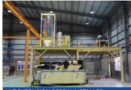
10 T EXTRUSION SCREW INSTALLED
