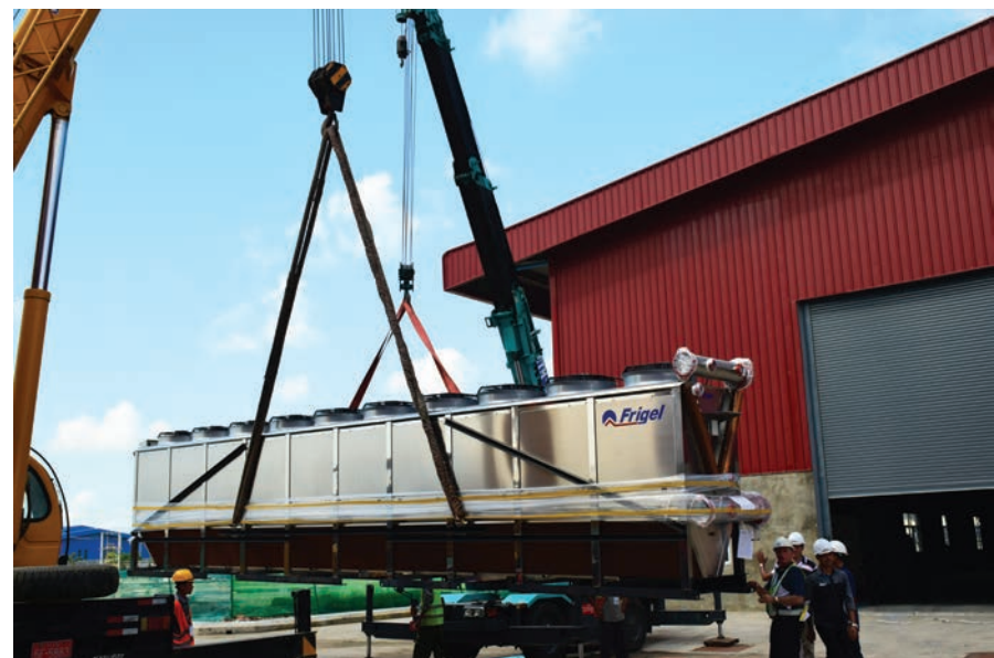
40FT HEAT EXCHANGER AWAITING ASSEMBLY OF LEG SECTIONS
