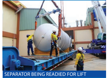
SEPARATOR BEING READIED FOR LIFT
