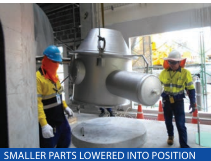
SMALLER PARTS LOWERED INTO POSITION
