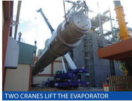
TWO CRANES LIFT THE EVAPORATOR
