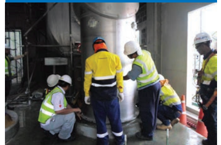
ALIGNING THE CHAMBER TO ITS BASE
