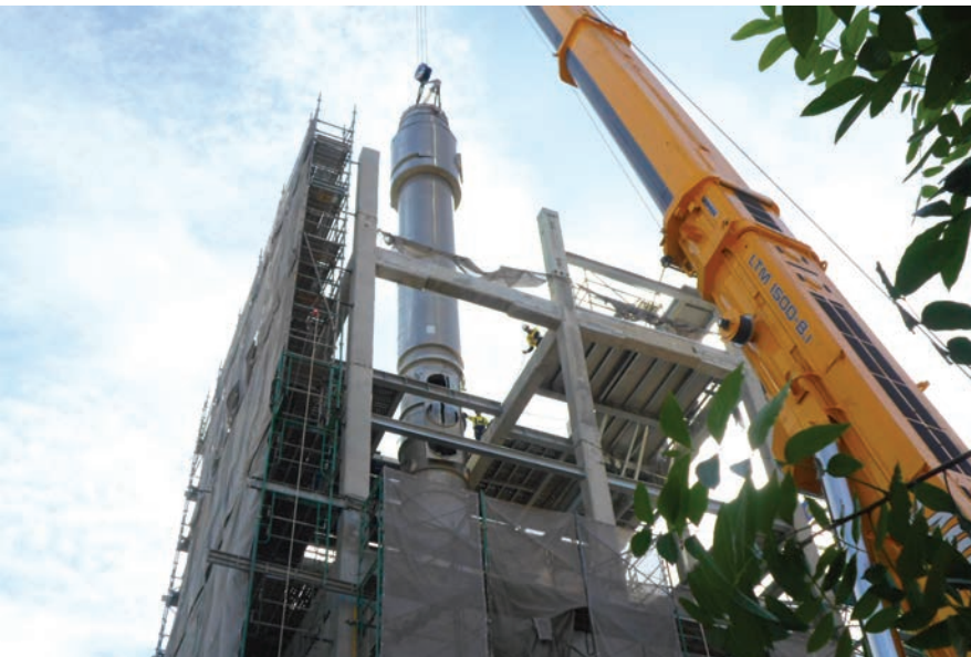
THE W100 28 TONNE EVAPORATOR CHAMBER IS CAREFULLY LOWERED INTO THE FACILITY
