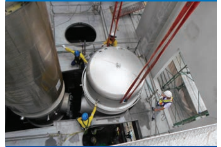
SEPARATOR LOWERED INTO POSITION
