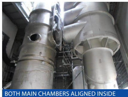
BOTH MAIN CHAMBERS ALIGNED INSIDE
