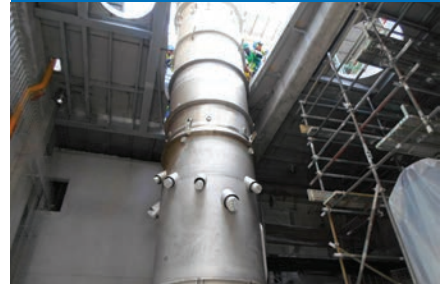
CHAMBER LOWERED THROUGH EACH FLOOR
