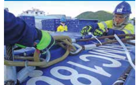
LIFTING SLINGS ATTACHED BEFORE PACKING
