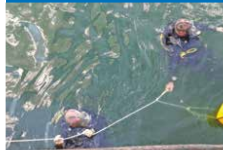
DIVERS ATTACHED THE SLINGS UNDERWATER
