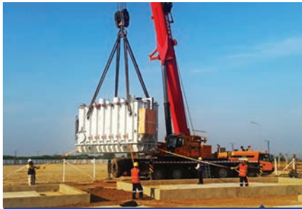
220 T CRANE PLACES THE TRANSFORMERS
