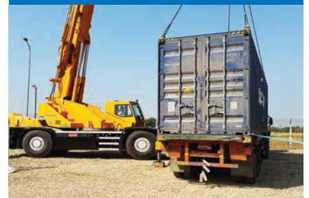
70 T CRANE UNLOADS SOC CONTAINERS
